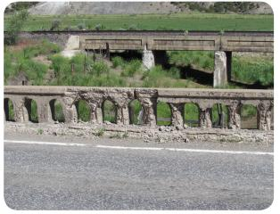
**Image 5.** Deterioration of the Deck on US 6 over Castle Creek in Eagle County (F-09-K)
